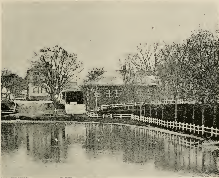
SCHOOL-HOUSE AT NORTHWESTERLY END OF BARTLET MALL.
